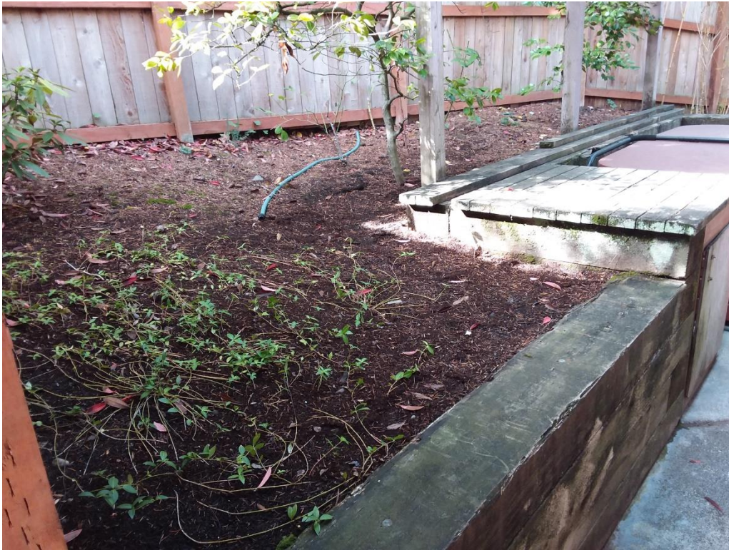
Figure 8. Looking at the landscape timber wall inside the fence.
